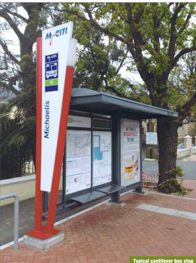
Typical cantilever bus stop
